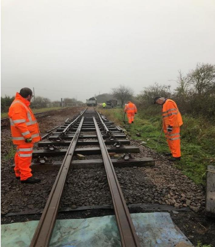
Moving On- On the last working day of 2020, a relatively small group of volunteers extended the track length by a further 60 feet, putting in place the next two full length rails seen below. Weighing in at just under 1 tonne per rail, a small team has to use ingenuity to ensure they keep a safe working environment and get the rails correctly placed in the sleeper chairs.
